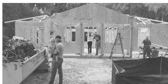
One of the houses FSC students helped build.
